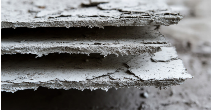
Detailed view of friable asbestos.
