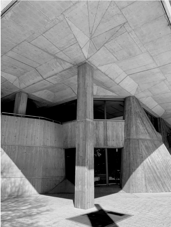
Henty House, Launceston, designed by Peter Partridge, Tasmanian Department of Housing and Construction. Image: David Beynon
