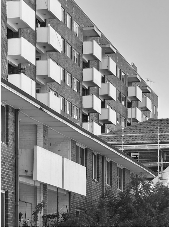
Wandana Flats north-east view from Coghlan Road. K. Hislop 2026
