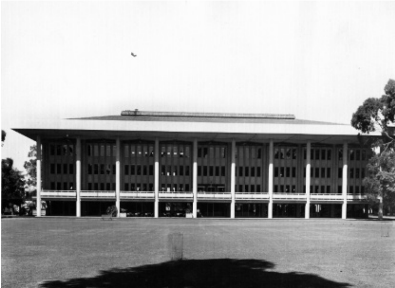
North elevation of the Reid Library. Image courtesy of the UWA Archives.
